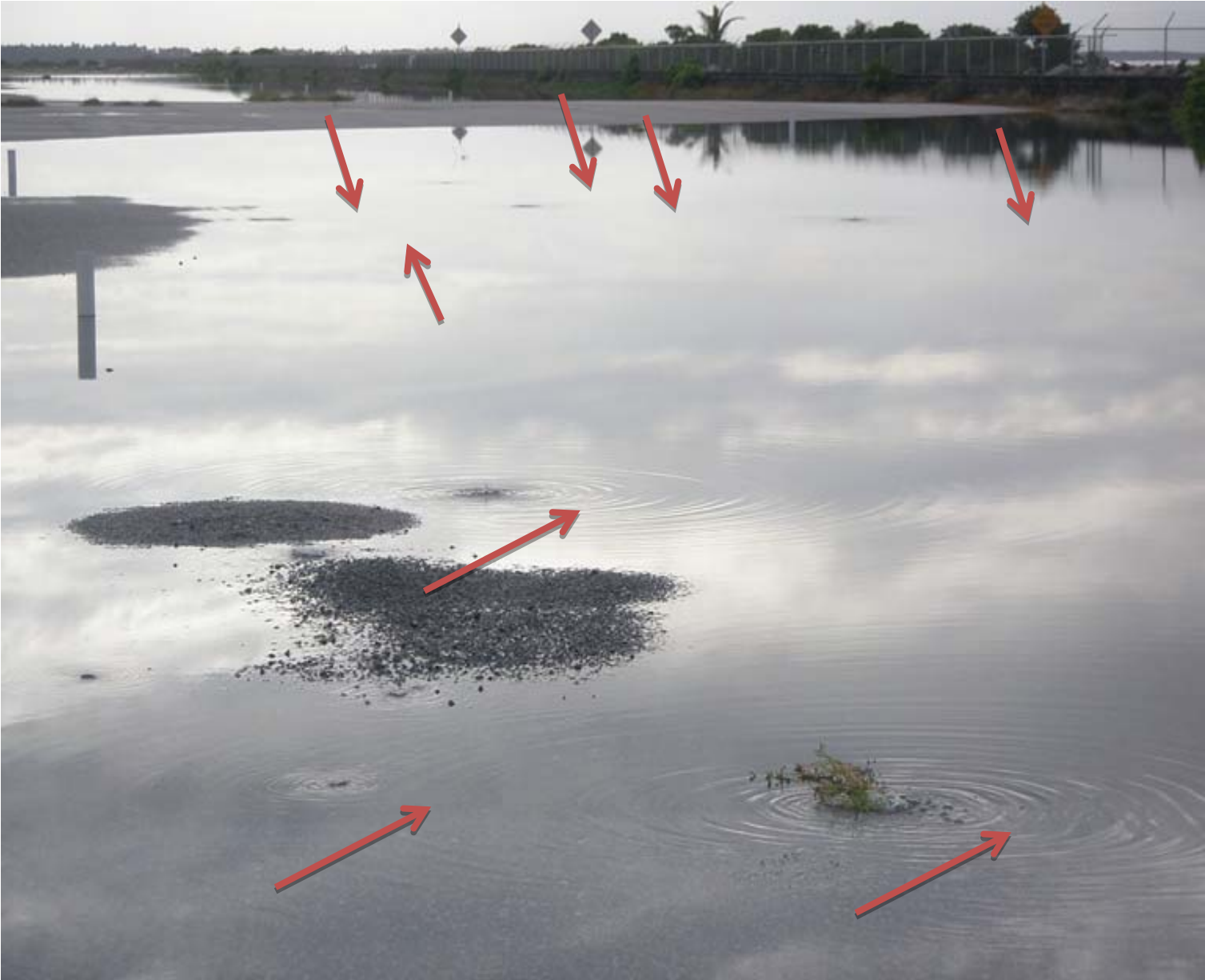
Multiple cracks with air bubbles coming through.
